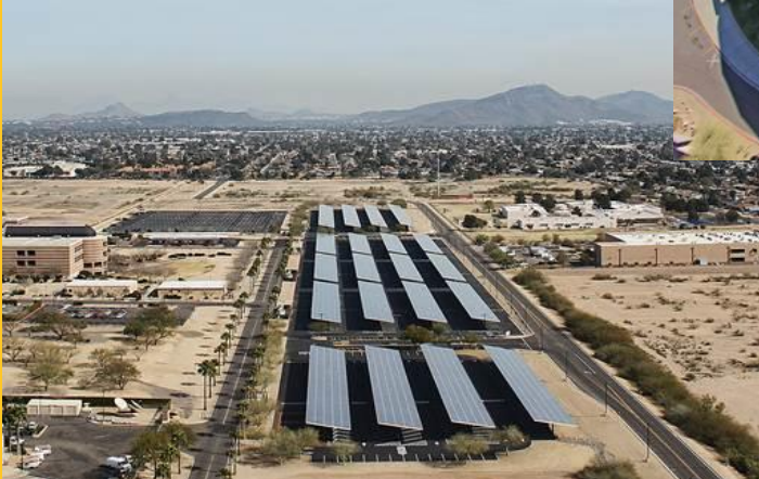
West Prkg, 2,680 kWdc, PV
