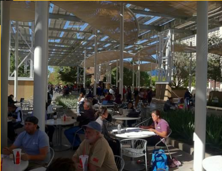
Orange Mall PP, 310 kWdc, PV
