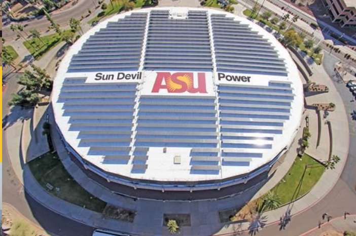
WFA, 497 kWdc, Fixed RT PV
