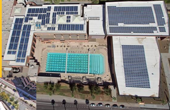
SDFCT, 1411 kWdc eq. (thermal) and 261 kWdc (Fixed PV)
