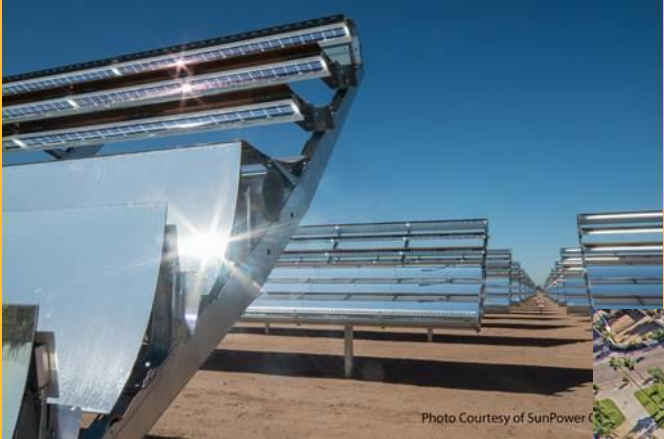
Sunpower c7, 1250 kWdc, SAT CPV
